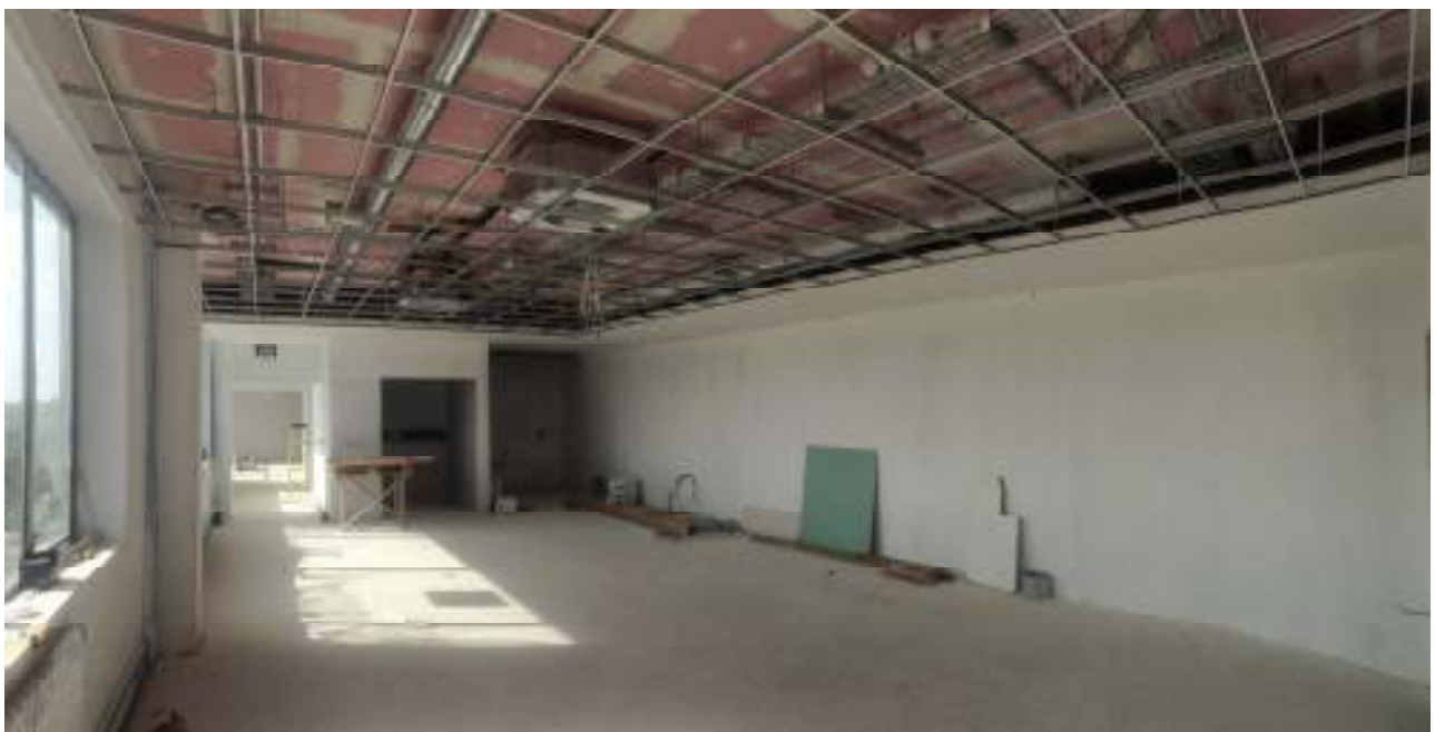
First Floor Office Area
