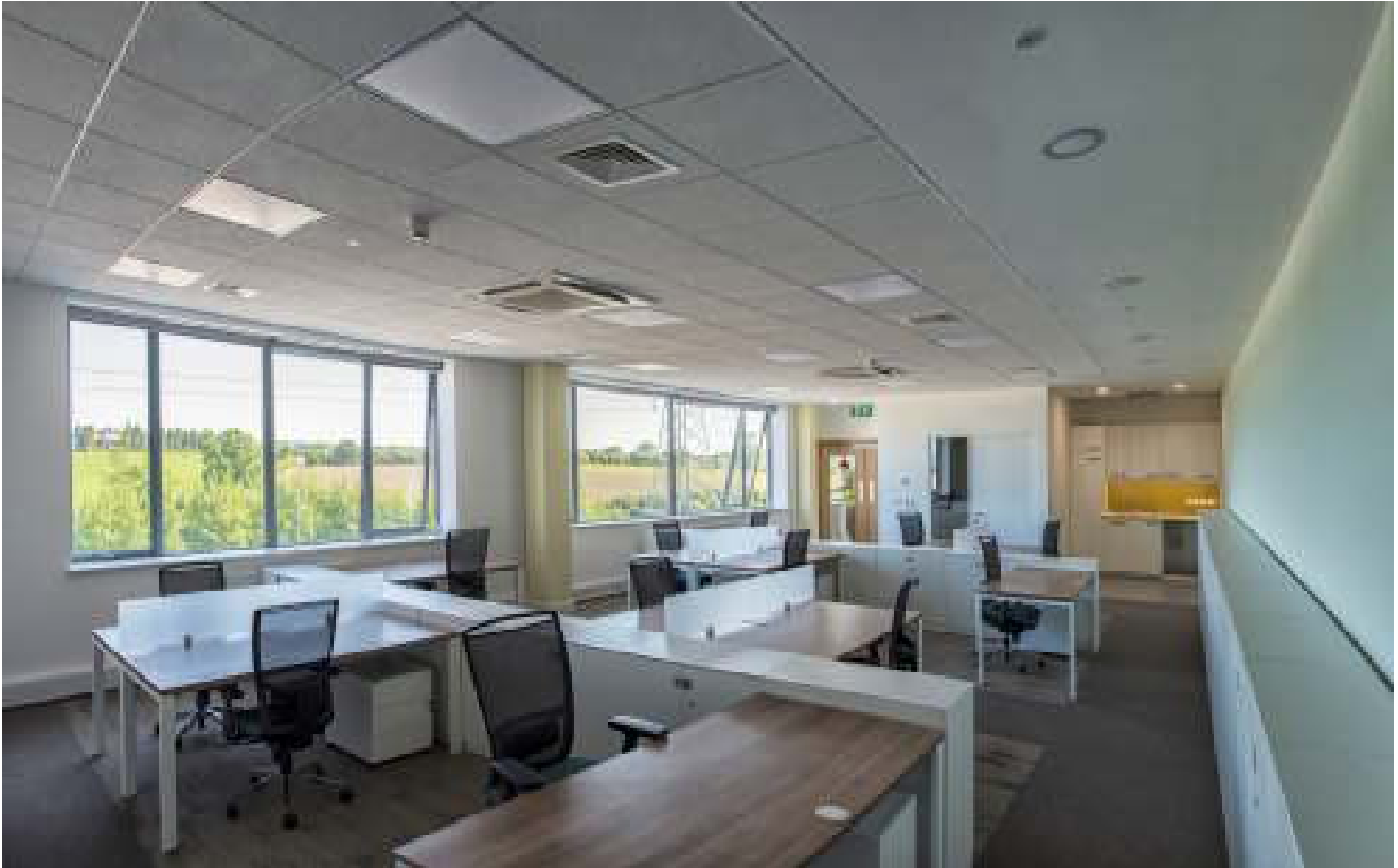
First Floor Open Plan Office Area
