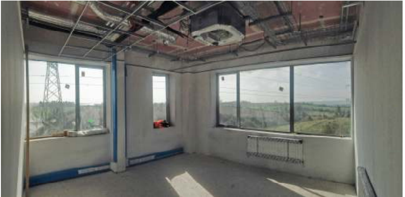
First Floor Office
