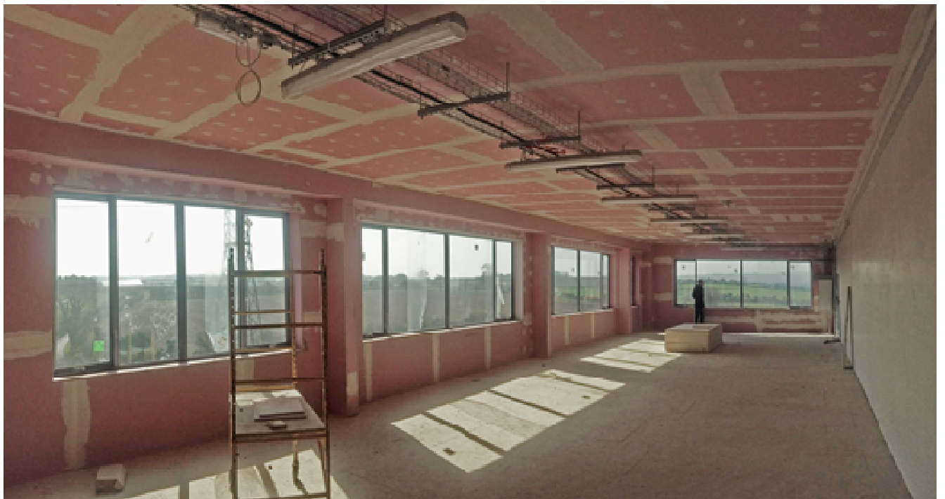
First Floor Office Area
