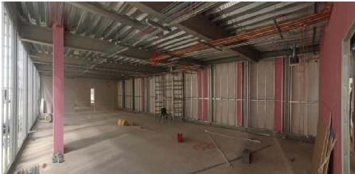
Ground Floor Office Area, new mezzanine floor over
