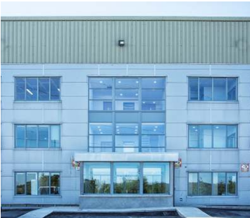
Front Façade, including new porch entrance with natural zinc cladding to match existing Kingspan Architectural metal cladding system
