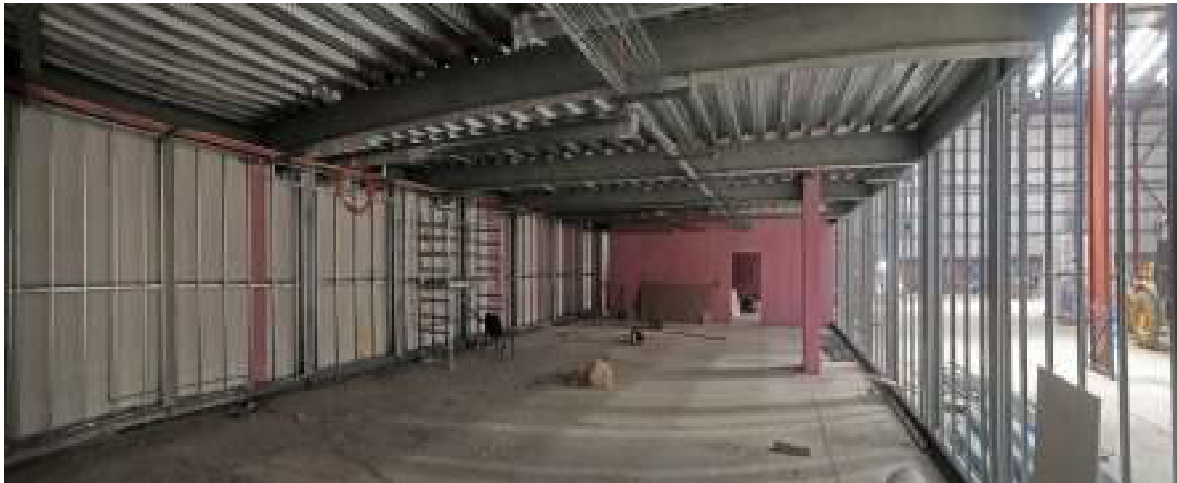
Ground Floor Office Area, new mezzanine floor over
