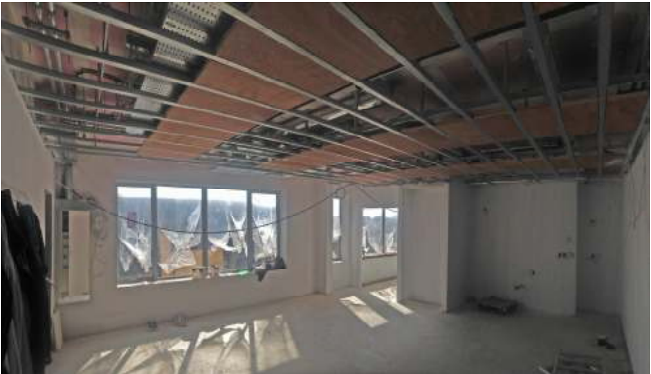
First Floor Office Area
