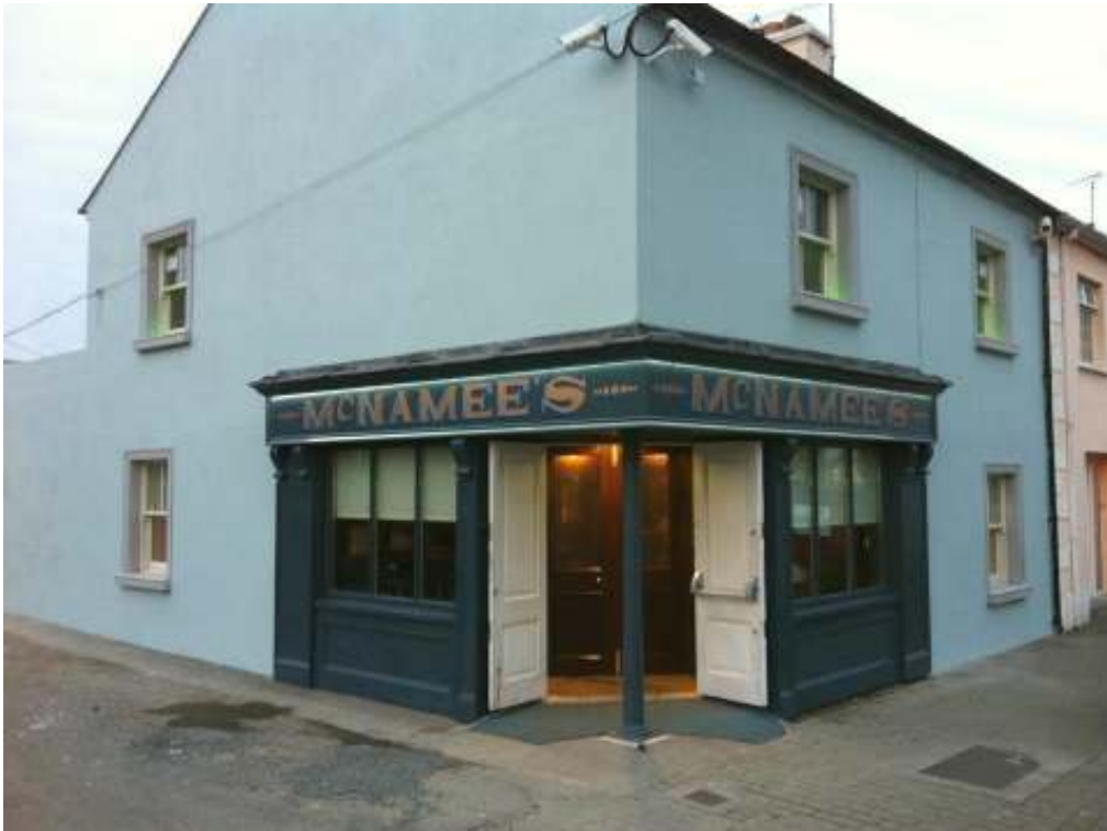
New corner entrance
