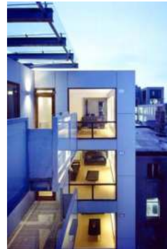
Upper floor apartments
