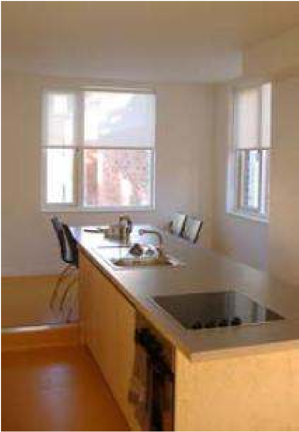
Kitchens units are bespoke birch ply doors and carcasses
