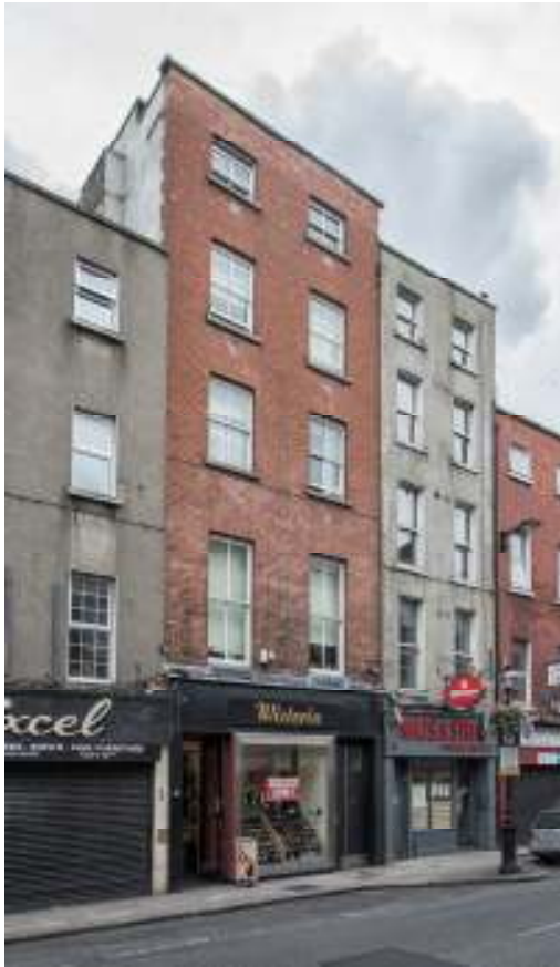
Front Façade – Capel Street
