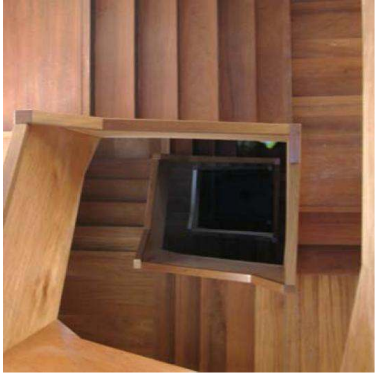
Timber clad, steel frame staircase
