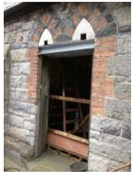
New structural Ope
