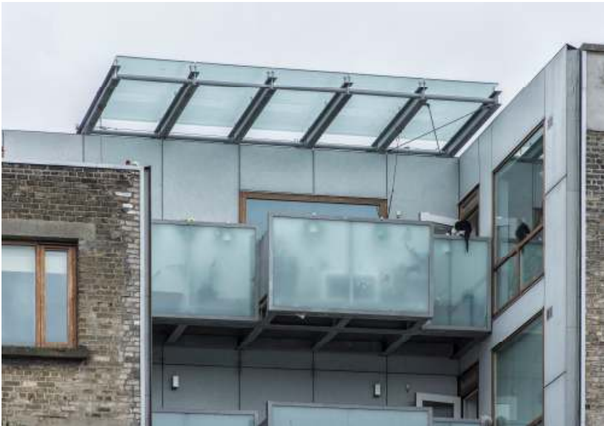
Detailed views of side elevation, featuring bespoke glazed balustrades, metal deck access with glazed canopy over and Tegral Pelicolor cladding
