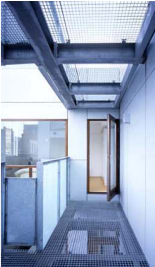
Metal deck access
