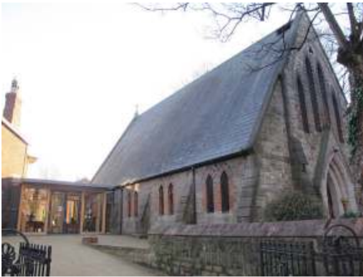
View from Adelaide Road
