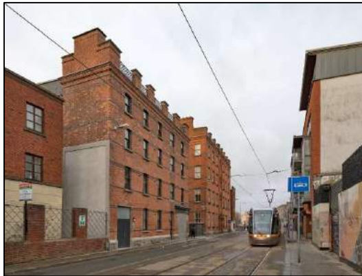
Looking West on Benburb Street
