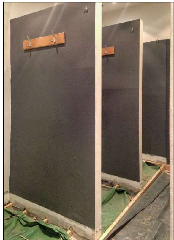
New partitions to changing rooms
