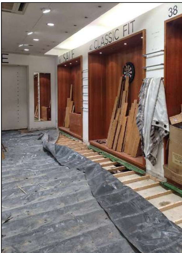
New subfloor to retail area
