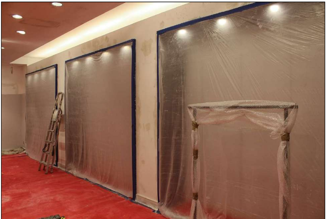
Dust proofing installed to storage areas
