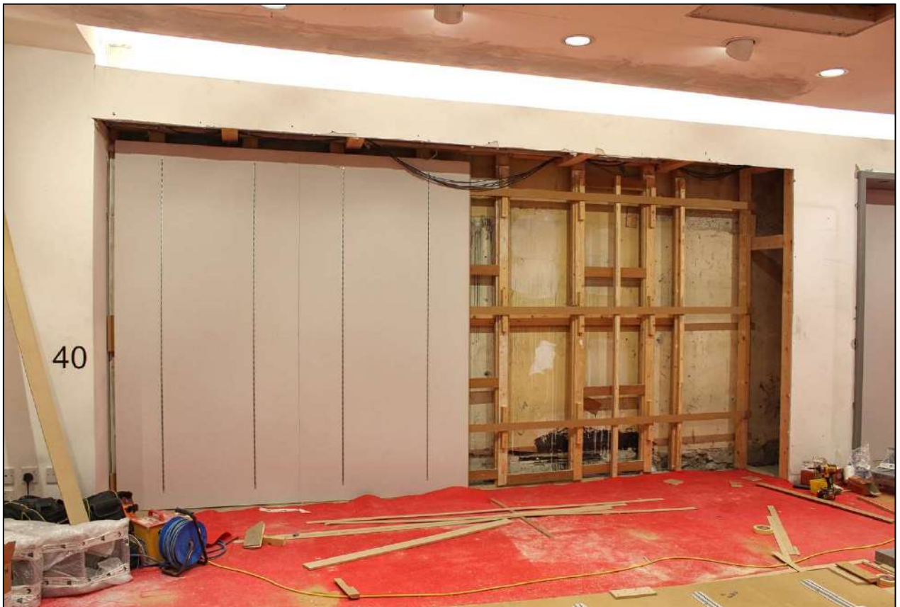
Protection to new flooring, completion of new storage areas
