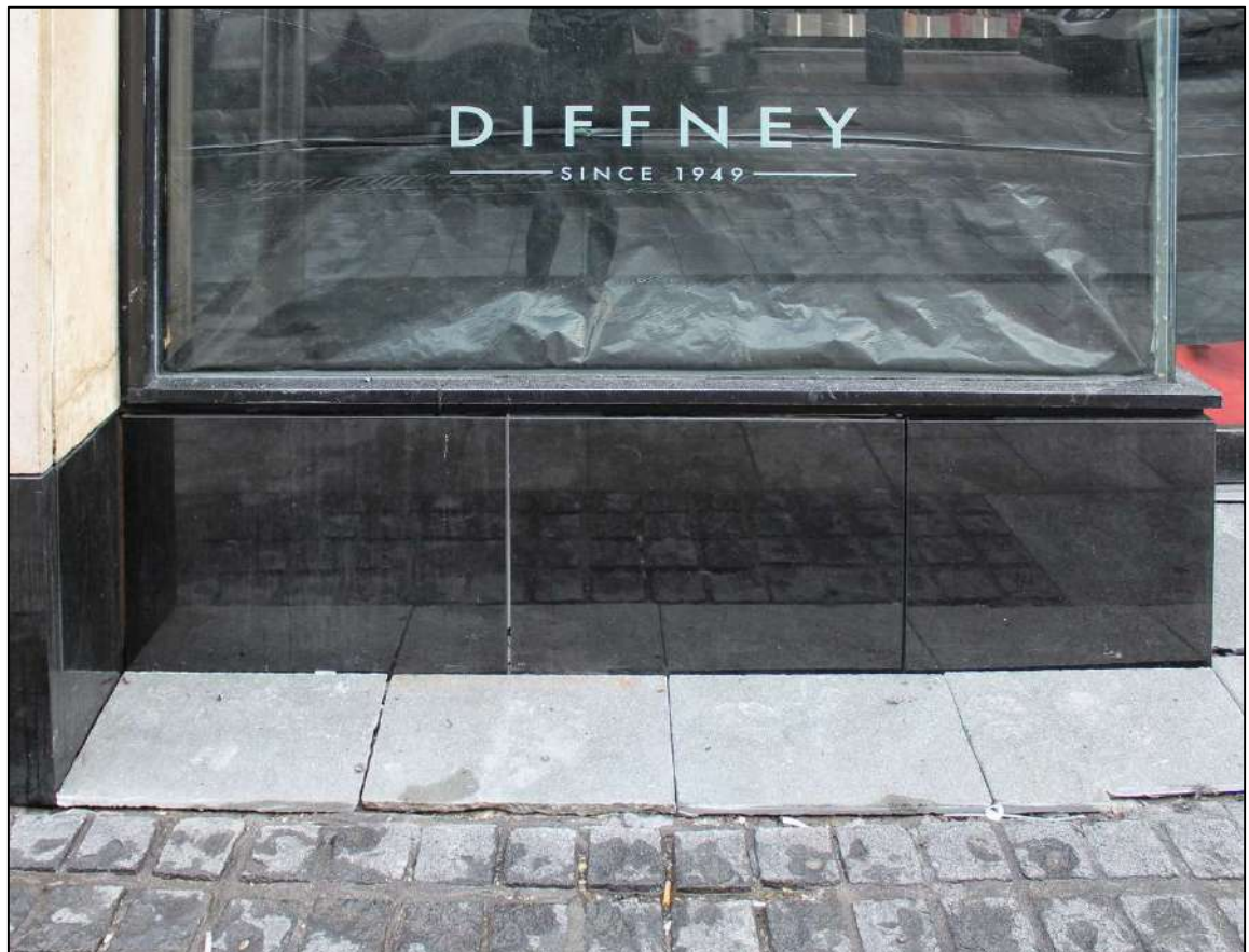
New stone plinth to shopfront
