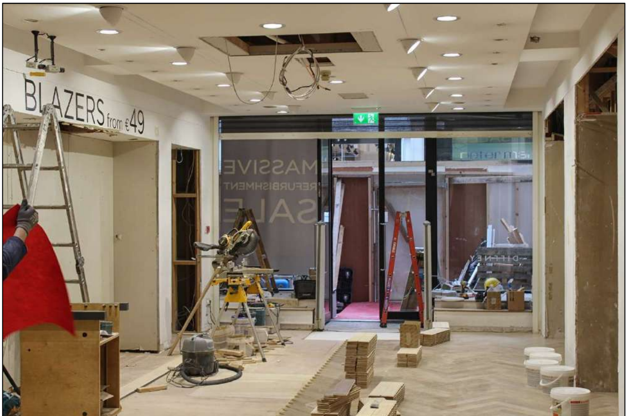
Laying of new herringbone hardwood timber flooring
