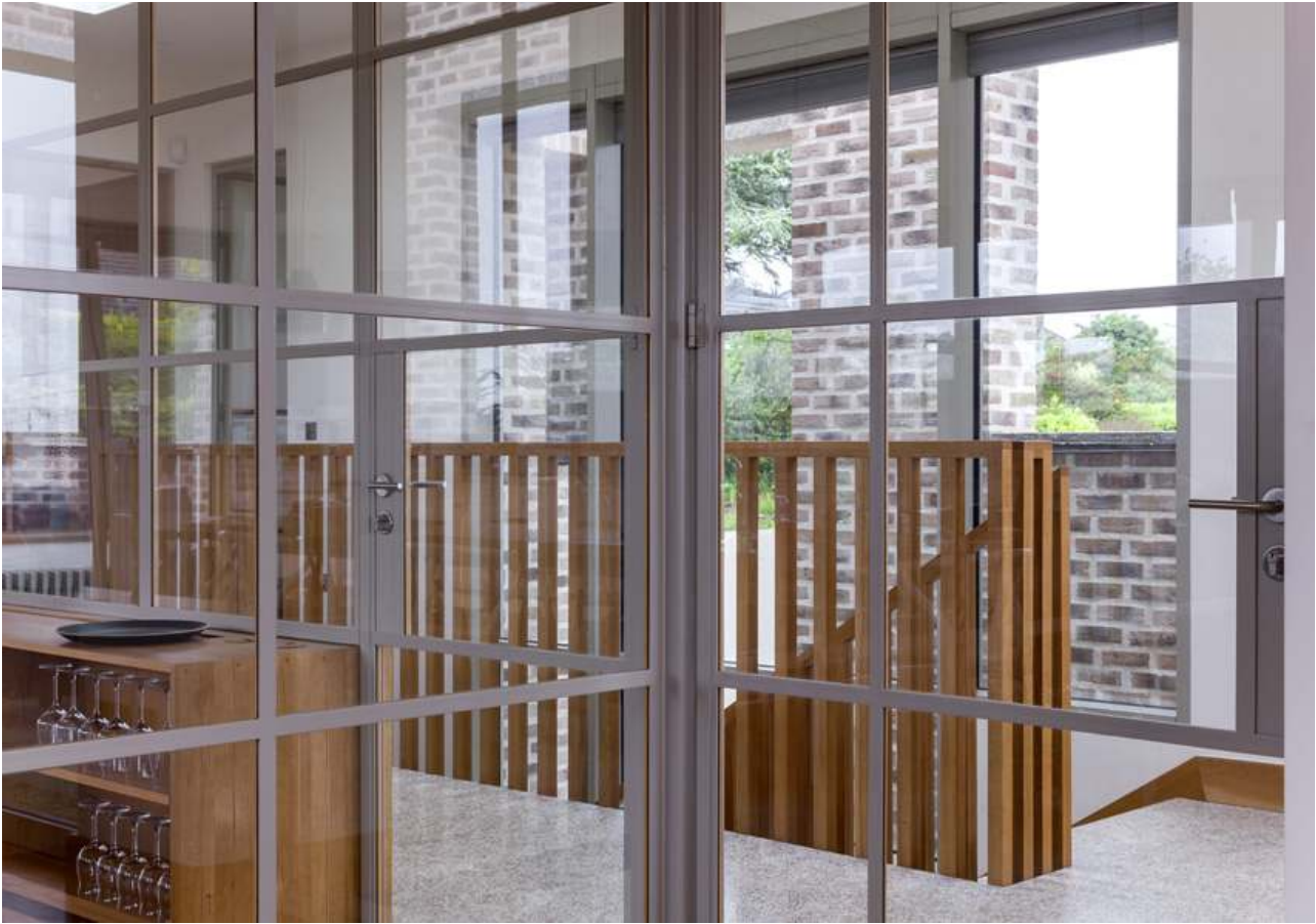
Bespoke internal glazed Crittal partitions
