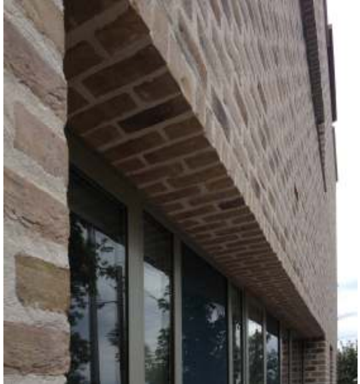
Side elevation, featuring 8 meter long window, 25mm joints with lime mortar, 35mm peps, natural slate cills and a brick-and-a-half hanging detail
