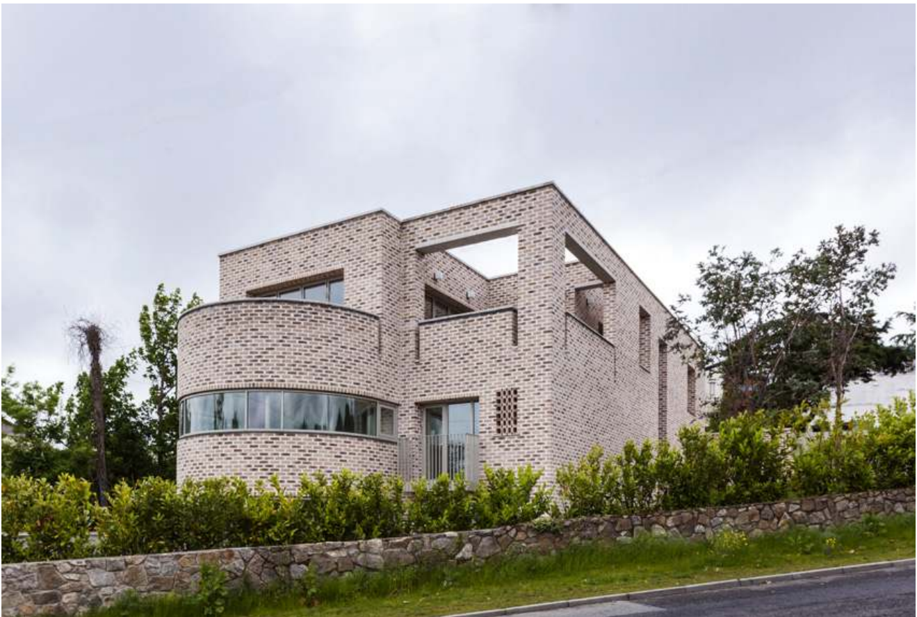
Side elevation, featuring 8 meter long window, 25mm joints with lime mortar, 35mm peps, natural slate cills and a brick-and-a-half hanging detail
