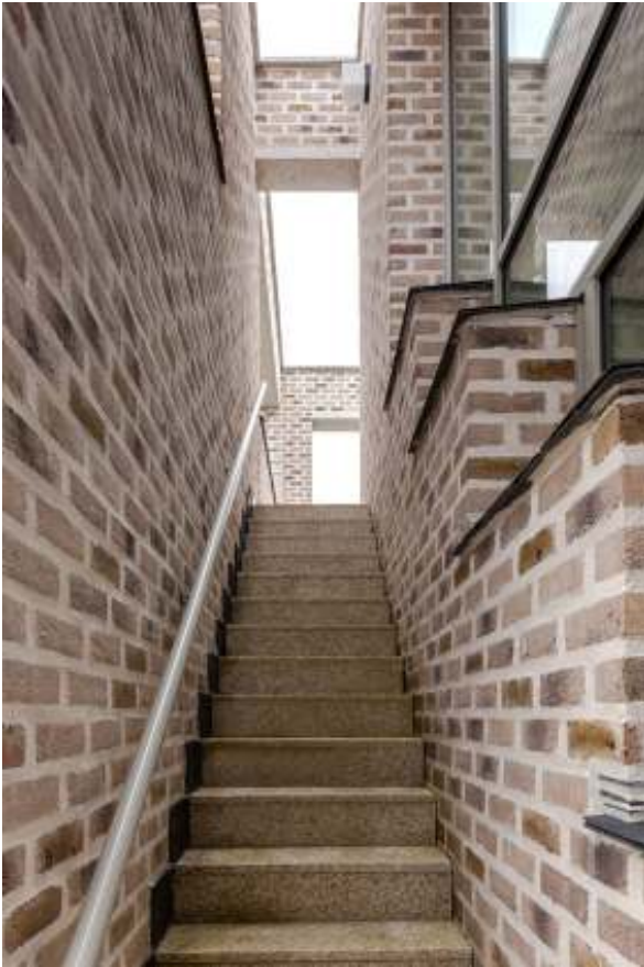
External Staircase, with natural slate cills
