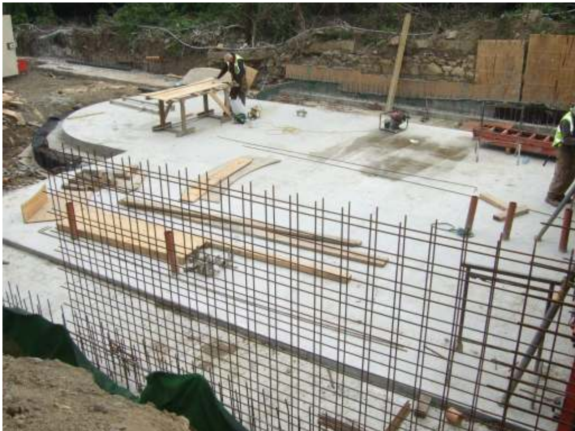
Installation of Concrete Reinforcing
