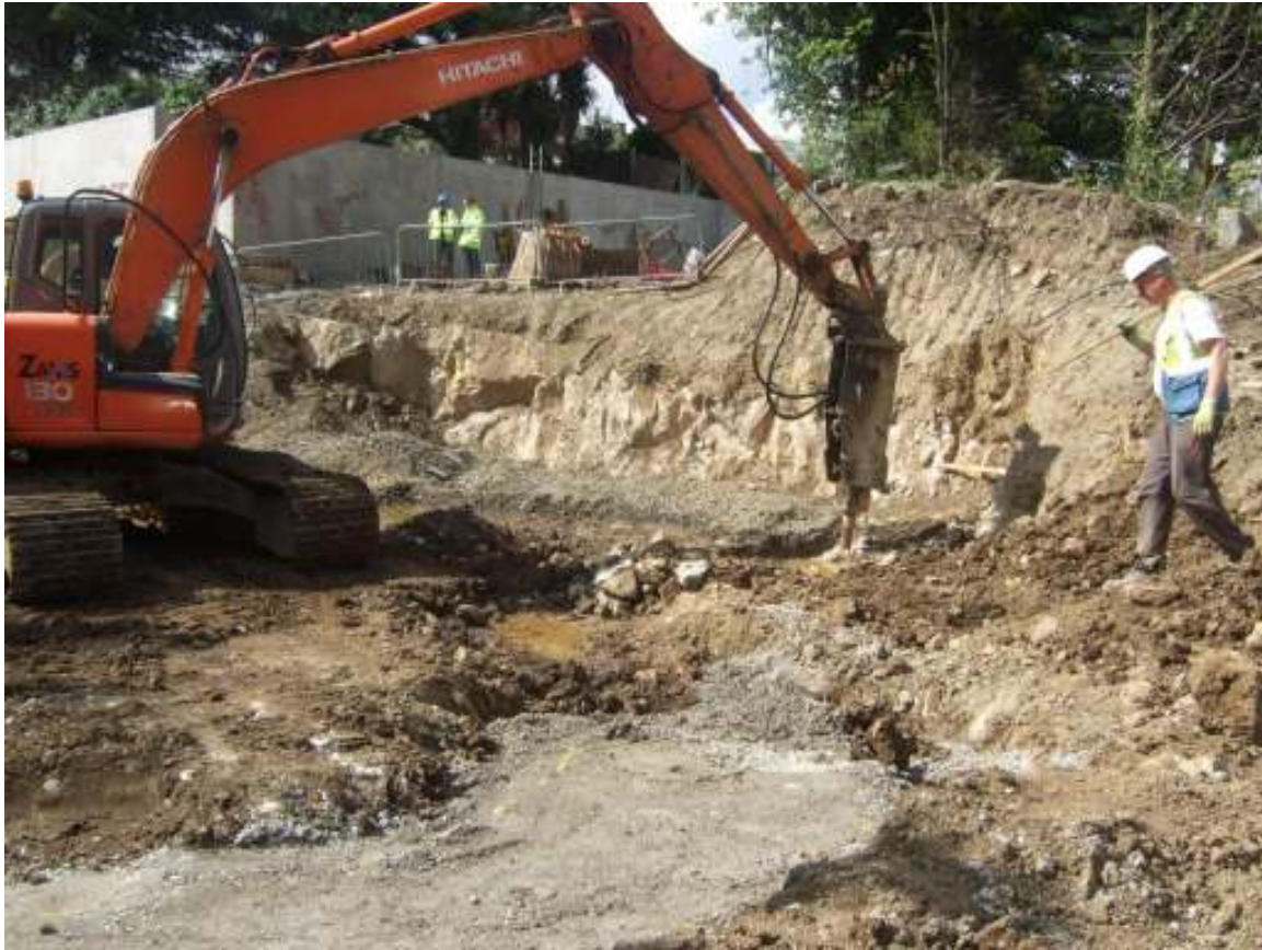
Excavations and Site set up
