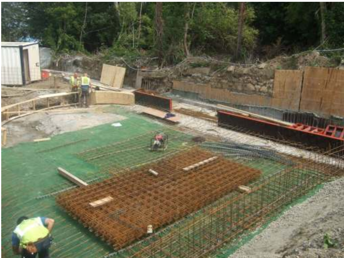
Installation of Concrete Reinforcement
