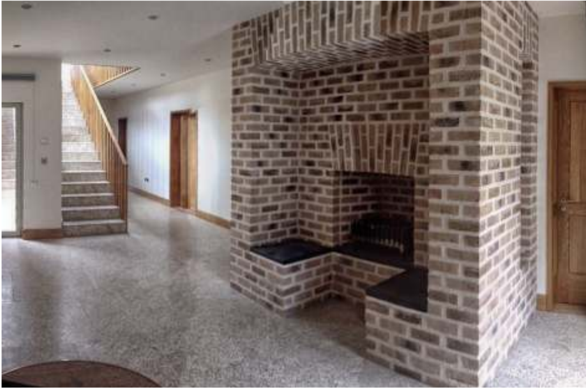
Solid fuel brick fireplace in entrance lobby, with Slivester buff polished granite floor
