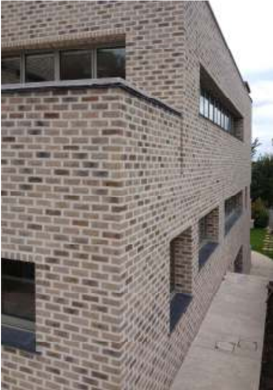
Side elevation, featuring 8 meter long window, 25mm joints with lime mortar, 35mm peps, natural slate cills and a brick-and-a-half hanging detail
