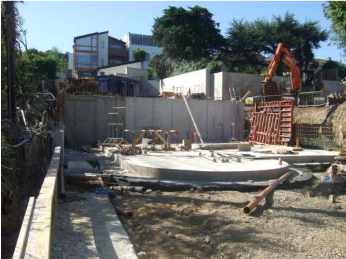
Basement Slab and retaining reinforced concrete wall
