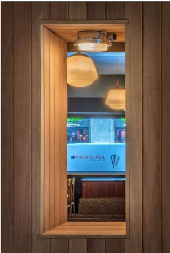
Bespoke timber cladding details to ground floor area
