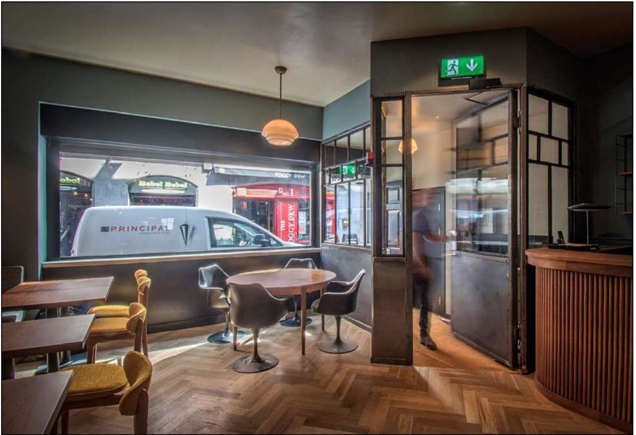
New bespoke, glazed, metal framed entrance lobby
