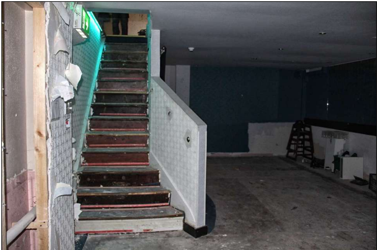
Existing unit prior to clearance
