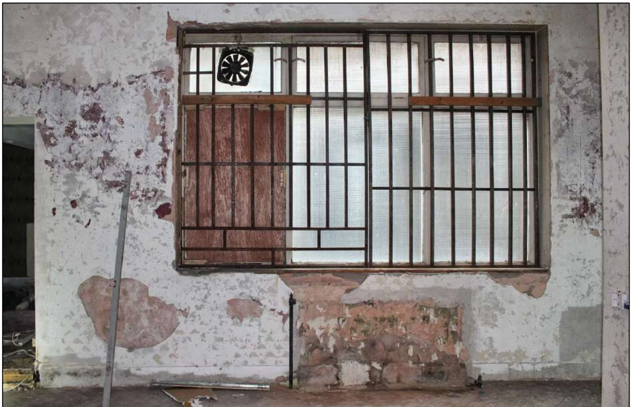
Preparation of Ground Floor for installation of new bar
