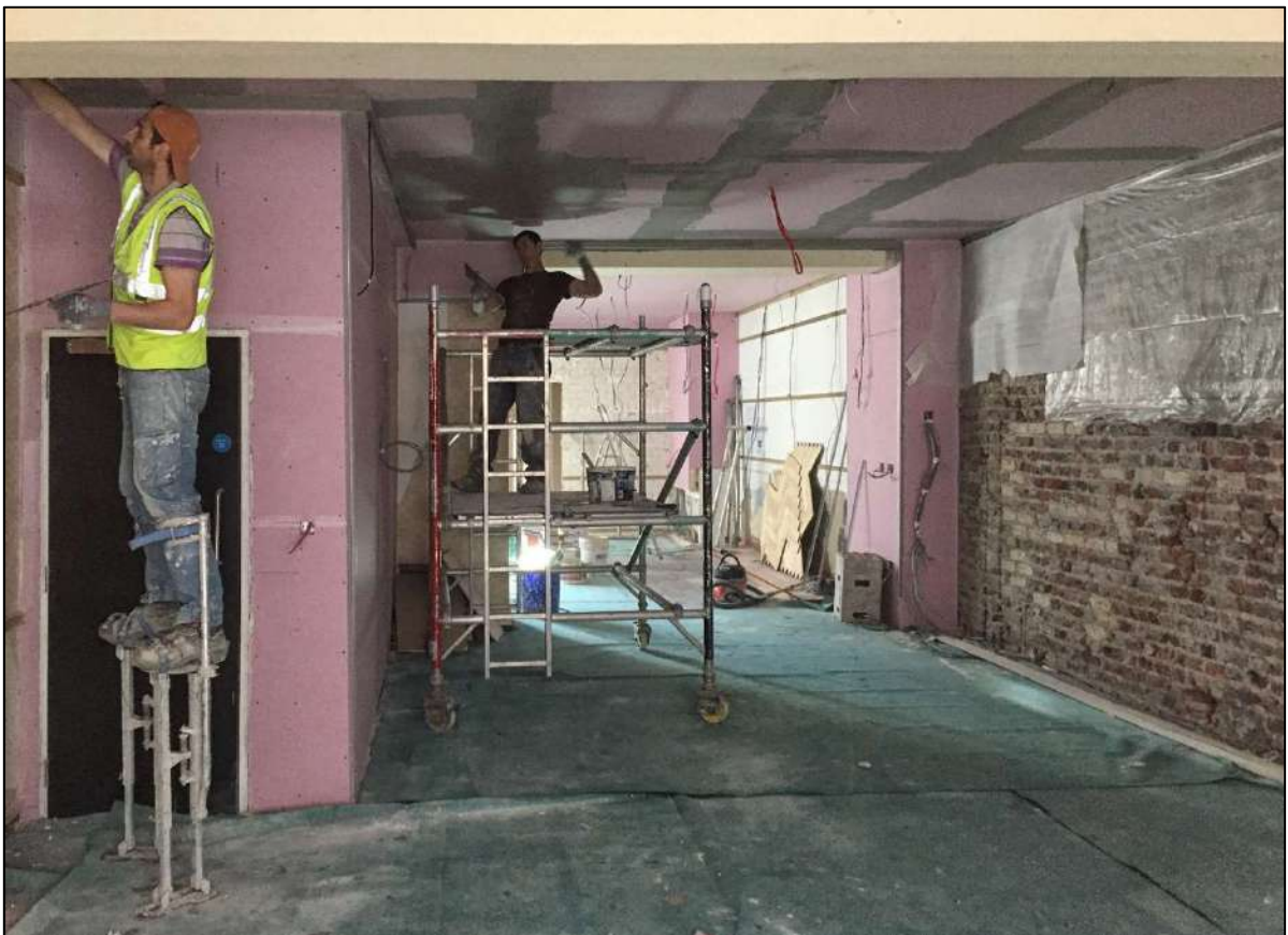
Commencement of plastering
