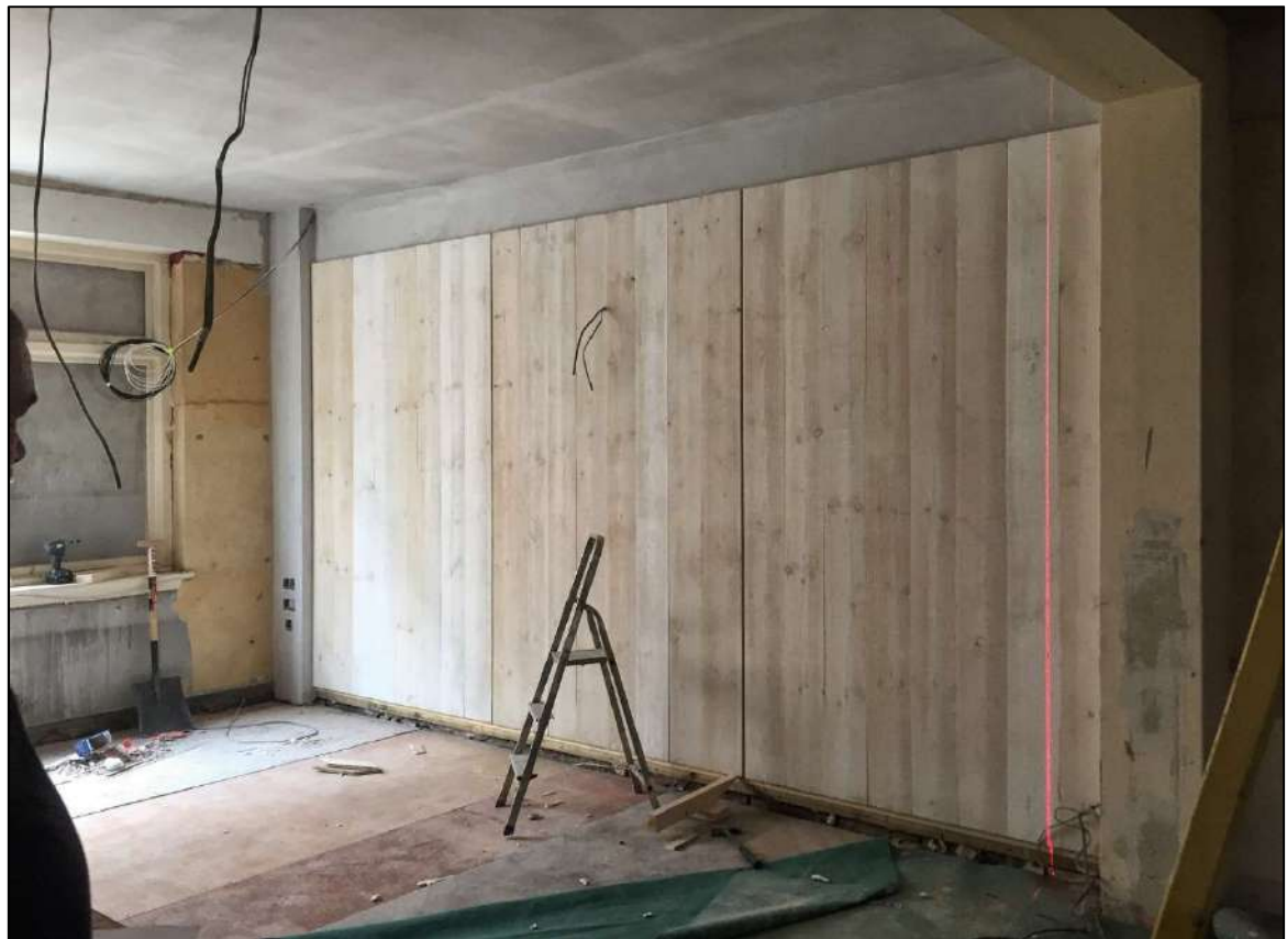
Installation of feature timber wall at first floor
