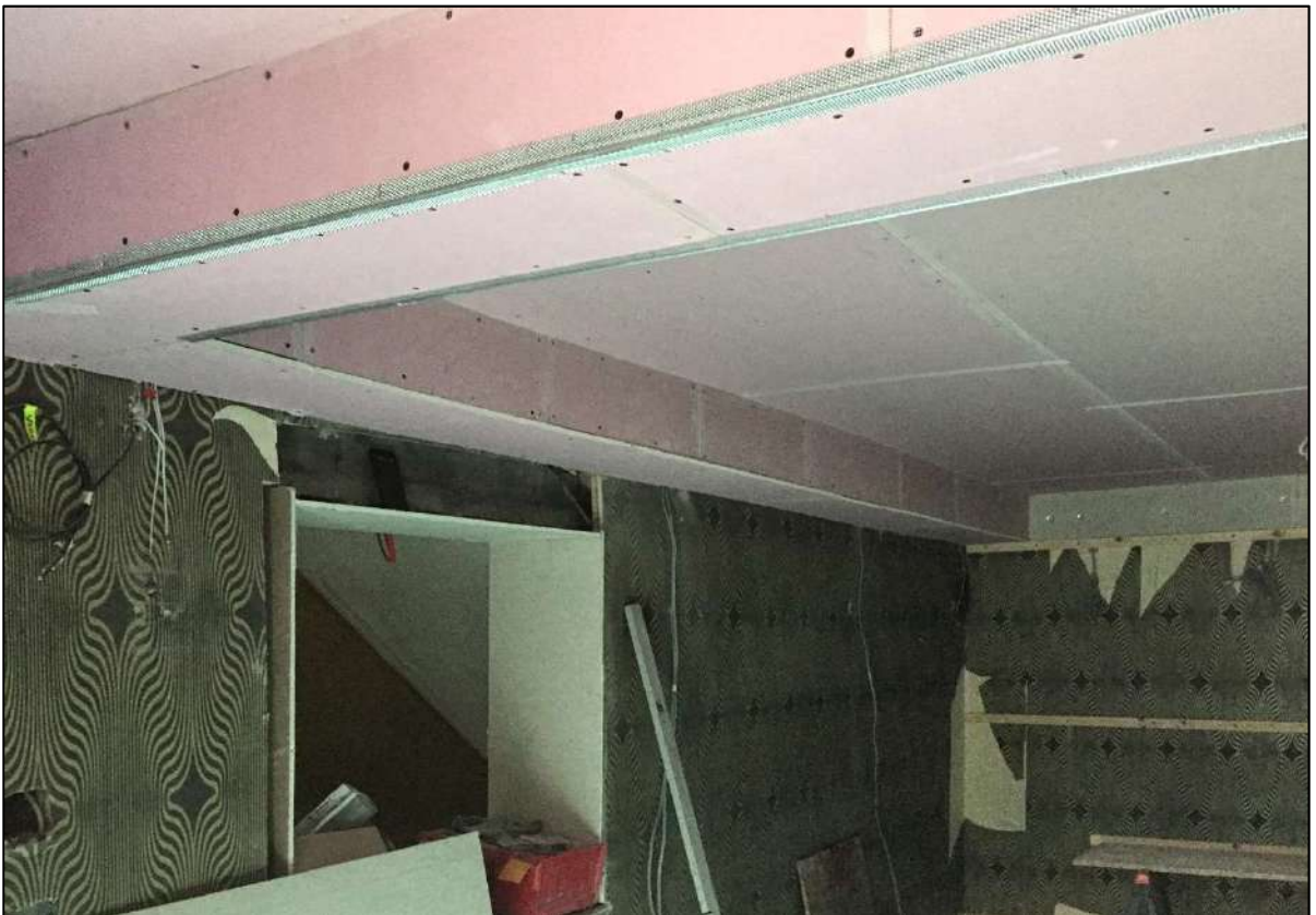
Installation of fire proofing between floors and around structure
