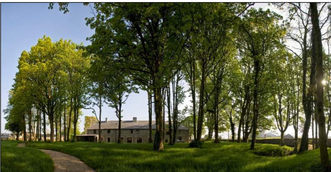
Clonabreany Courtyard post restoration and refurbishment
