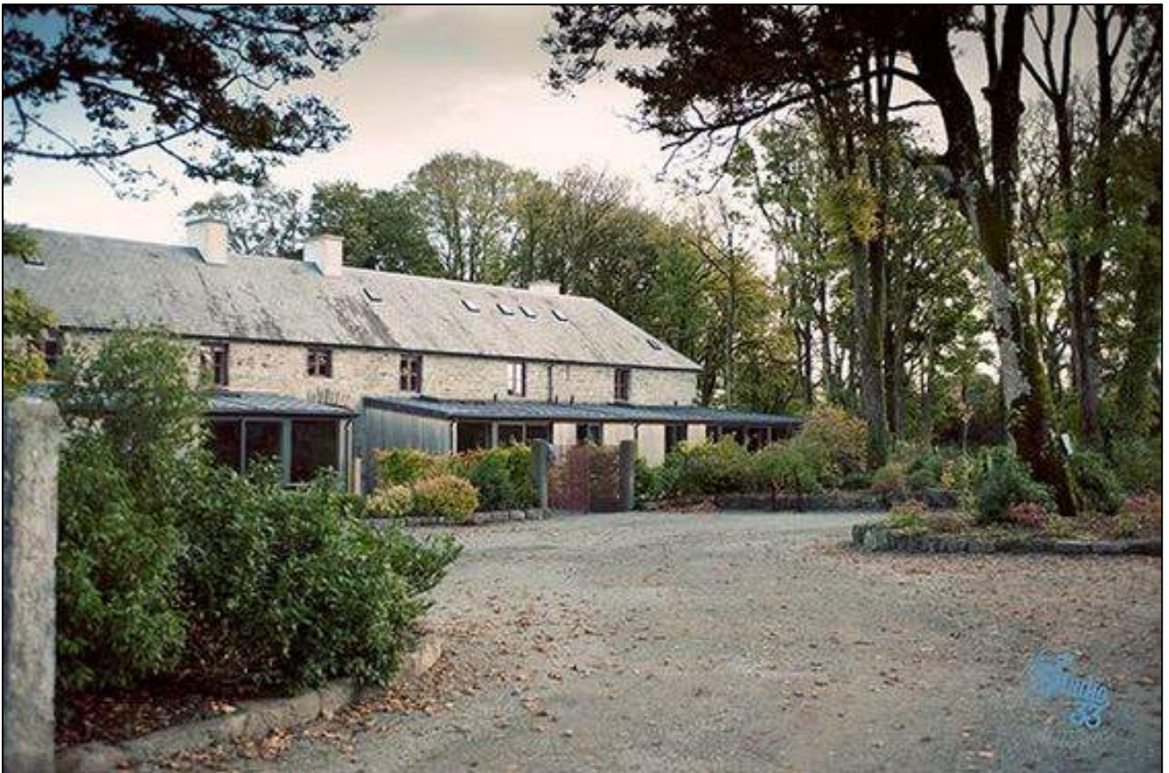
Clonabreany Courtyard post restoration and refurbishment
