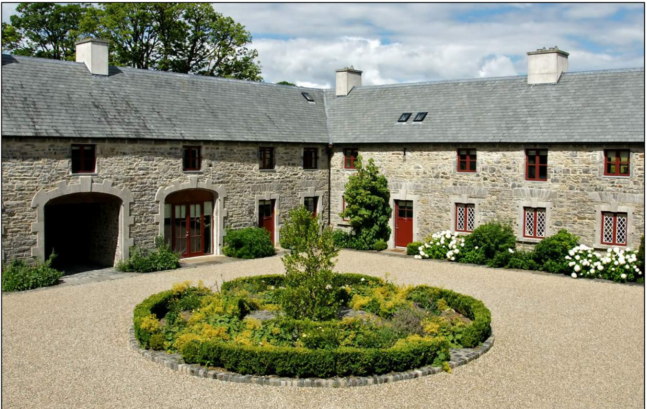
Clonabreany Courtyard post restoration and refurbishment
