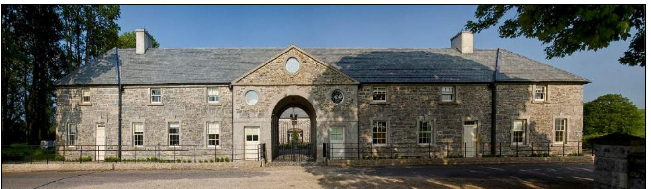
Clonabreany Courtyard post restoration and refurbishment
