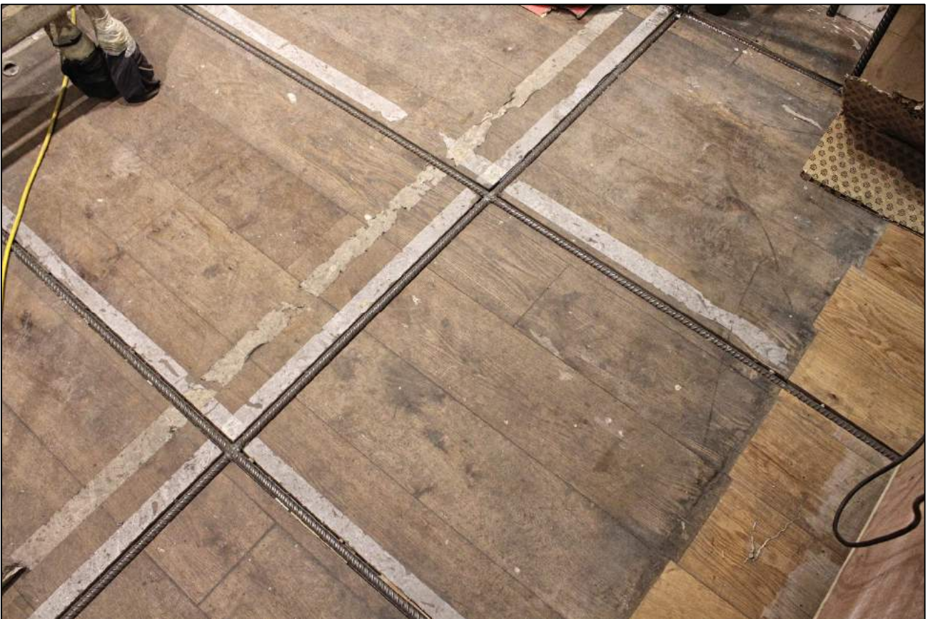
Various details: note rebar inset into existing timber floorboard
