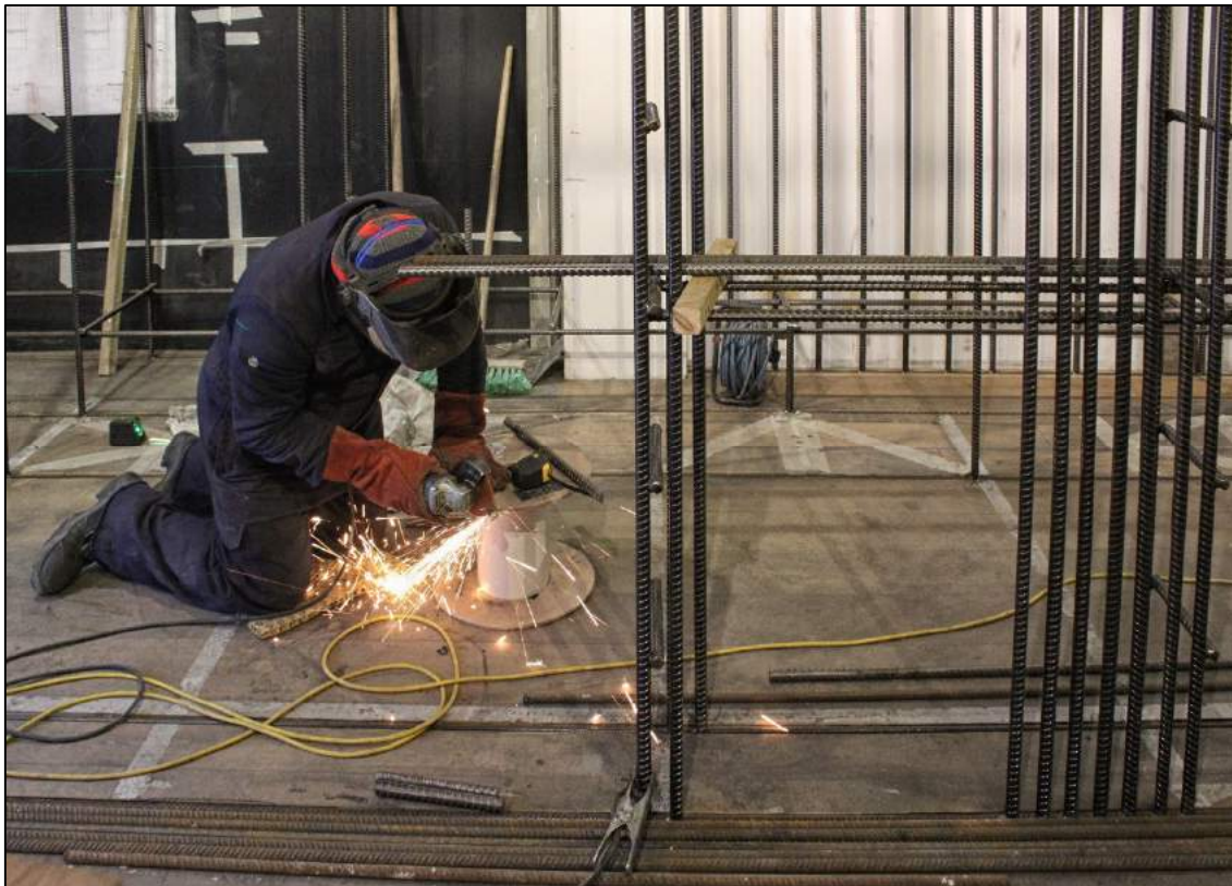
Installation of rebar throughout interior
